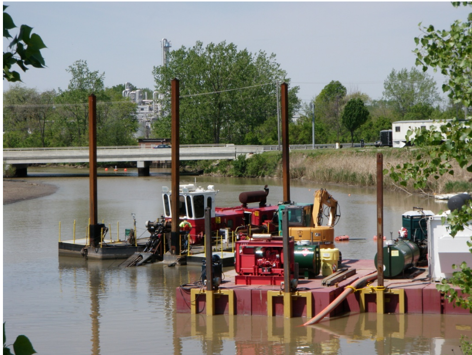
Figure 2. Ten-inch hydraulic dredge working area in Reach 2
