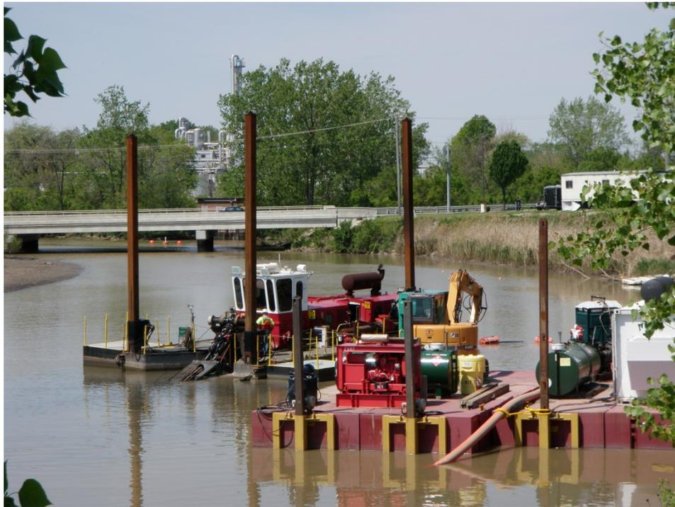
*Figure 2.* Ten-inch hydraulic dredge working area in Reach 2
