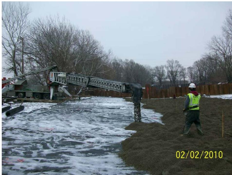
*Figure 1.* Granular cap placement by belt conveyor
