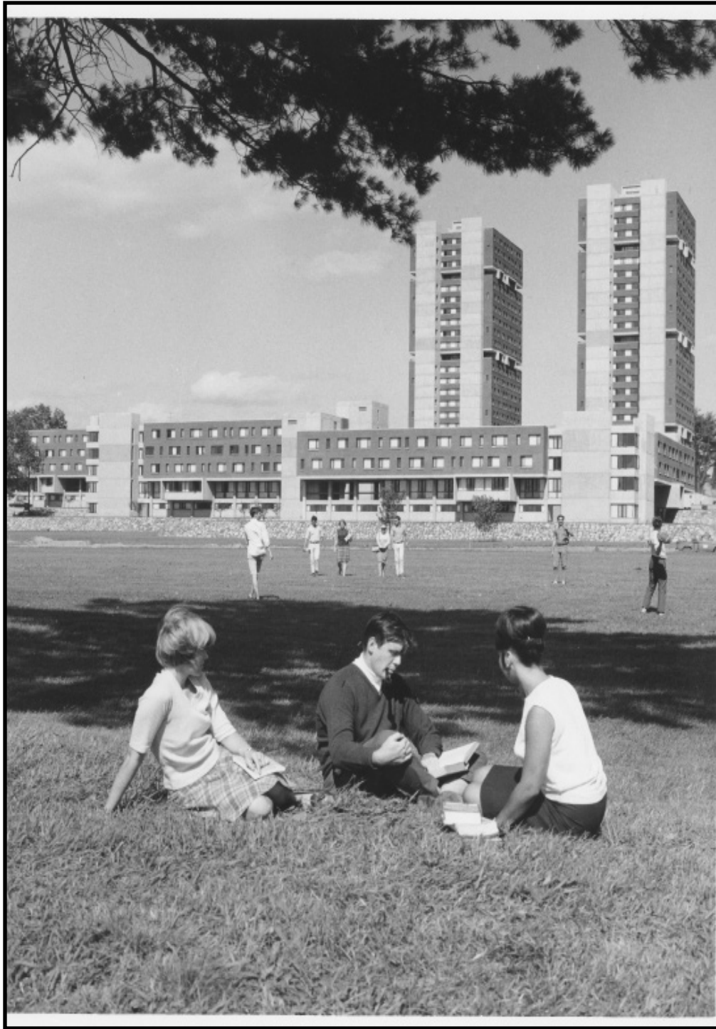
Southwest Residential Area, undated. University Photograph Collection (RG 110-176). Special Collections and University Archives, University of Massachusetts Amherst Libraries
