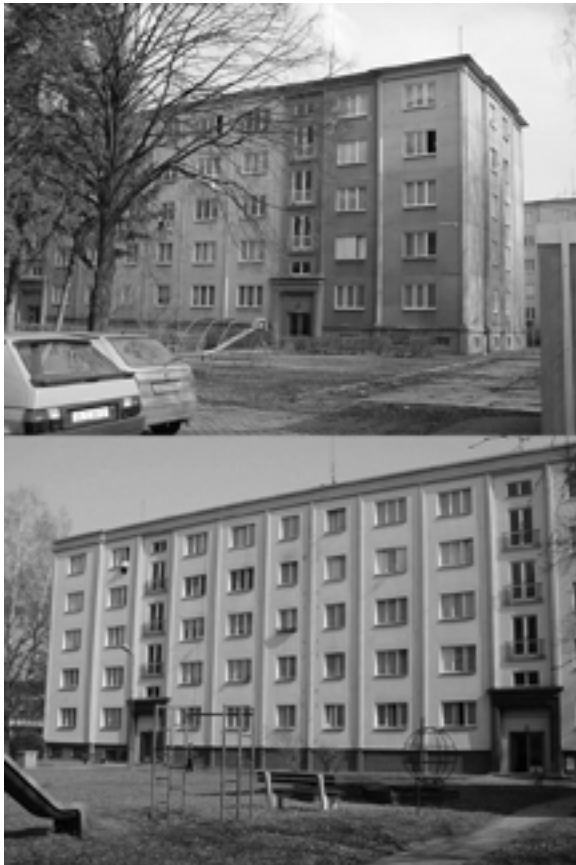
Fig. 3. Early Structural Panel Buildings in Zlín by Bohumír Kula and Hynek Adamec, 1954. Example before renovation (top) and example after renovation (bottom).
