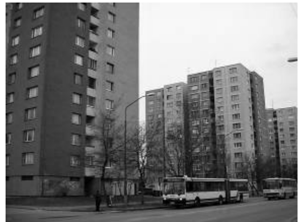
Fig. 4. Structural Panel Buildings in Petržalka neighborhood of Bratislava, Slovakia in 2003. Renovations were done on the building in front.
