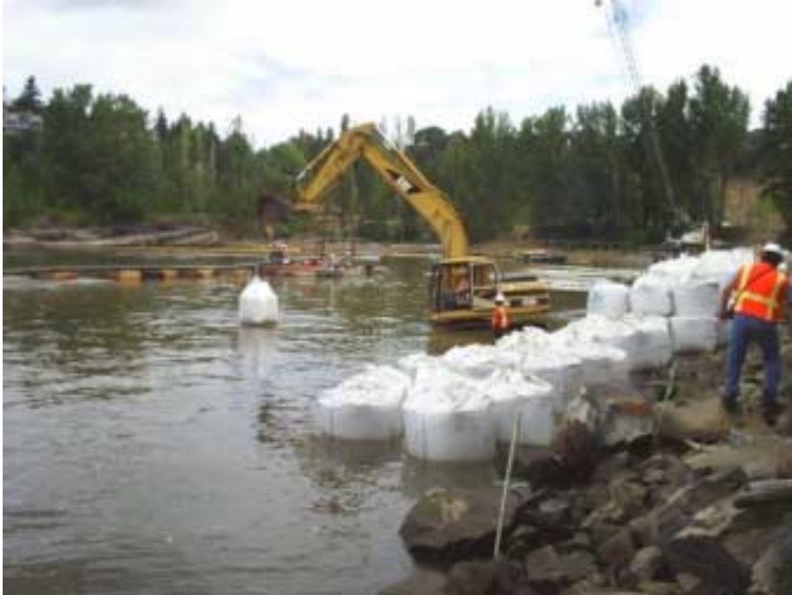
Figure 1. Deployment of Organoclay Cap at Willamette River
