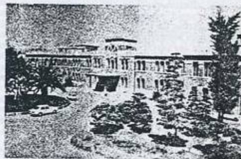
Administration Building, Kyushu University
