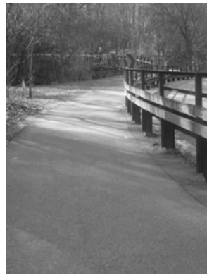
Figure 4. Example 2 of Co-Aligned Trail and Roadway Condition
