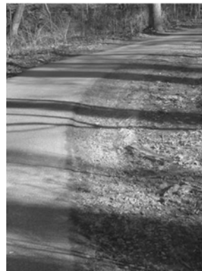
Figure 6. Conventional Off-Trail Raingarden Site Condition
