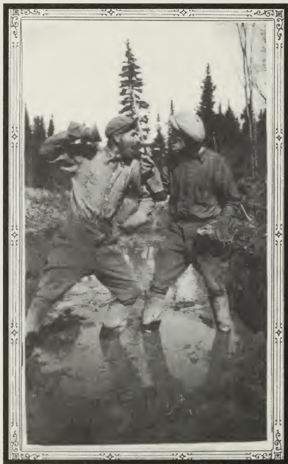
Harry Digging Ditches #3
