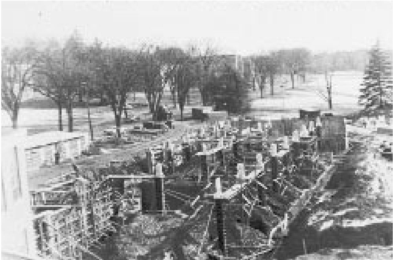
Construction of the Hasbrouck Addition, ~1962
