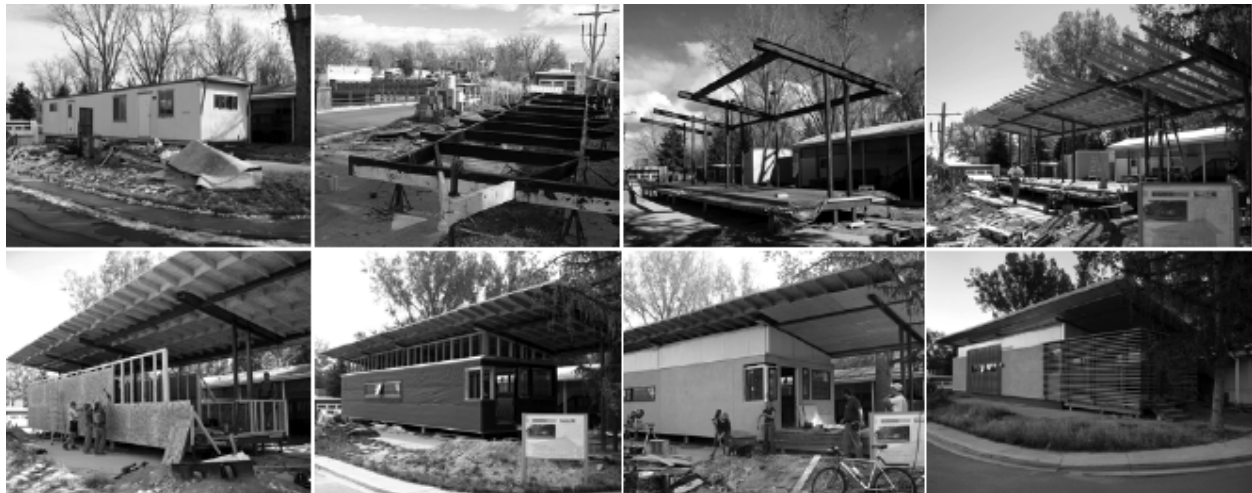
TrailerWrap: Transformation from stripped trailer chassis to affordable home
