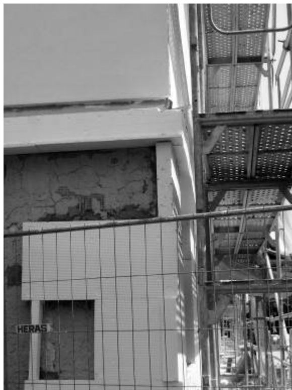
Fig. 5. Building in Brno undergoing façade renovation in 2006.
