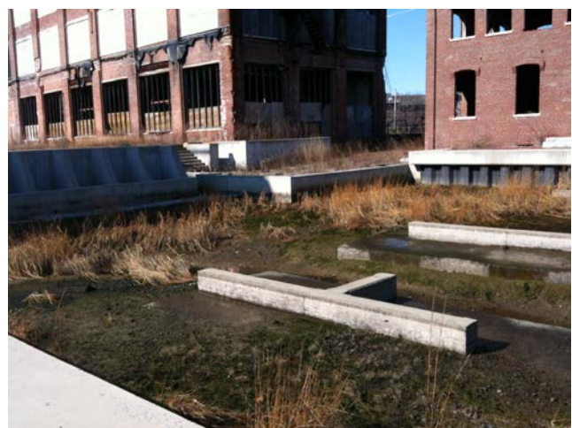
Canal system. Note the concrete bottom that was to be used in the skywalk development. (above) Area where canal water and river water would mix and overflow into the brackish pond. (below) Source: M. Iarossi
