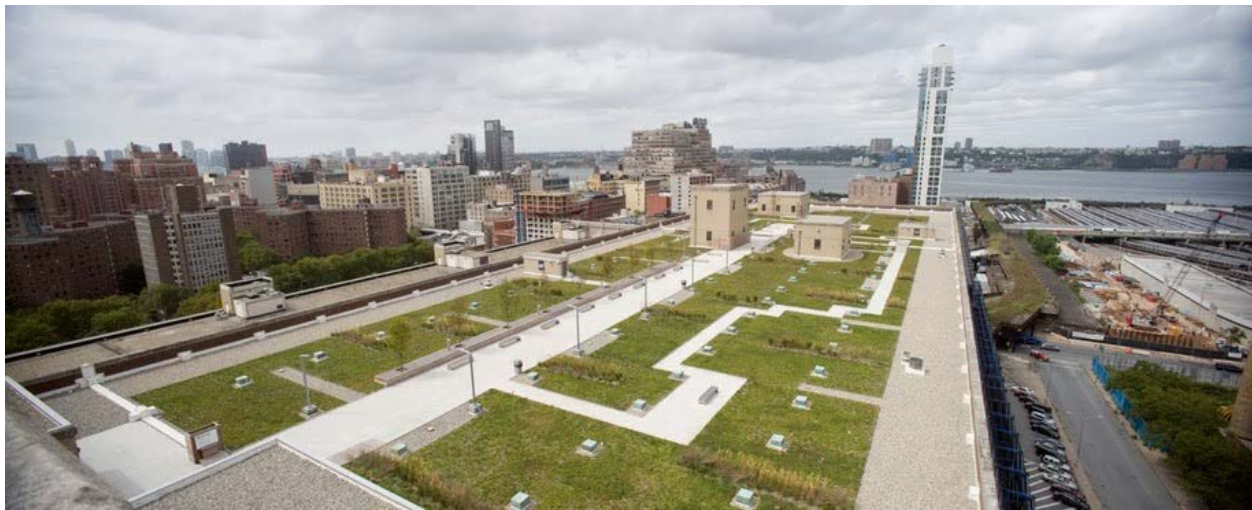
Fig. 2 Though this green roof is located on the U.S. Postal Service’s distribution facility in New York City, the size and shape are very similar to most mill buildings: massive and rectangular. This green roof decreased runoff by 75% during summer, saves $30,000 a year on energy costs and has a life span of about 50 years. Similar green roofs can be designed on mill structures. (Source: electrictreehouse.com )
