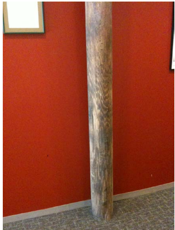
An original wooden structural beam that was preserved in redevelopment.
