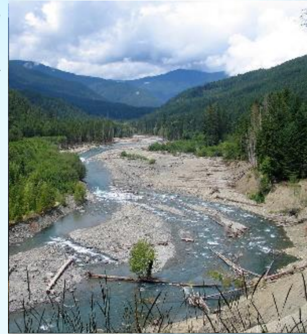
GLINES CANYON DAM, WA
