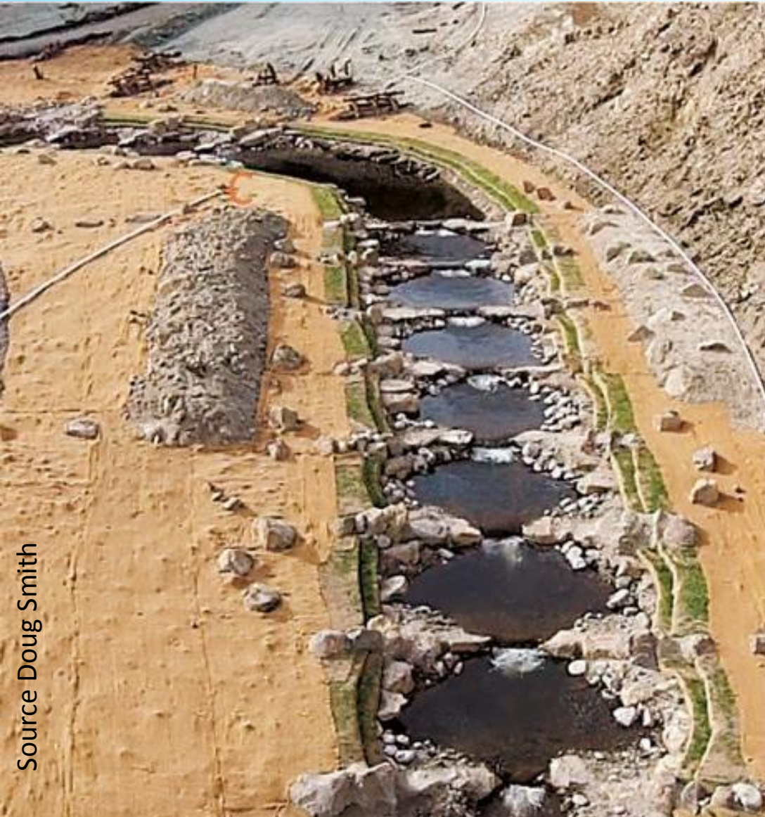
(Left) step pools were engineered in 2015 to last for decades
