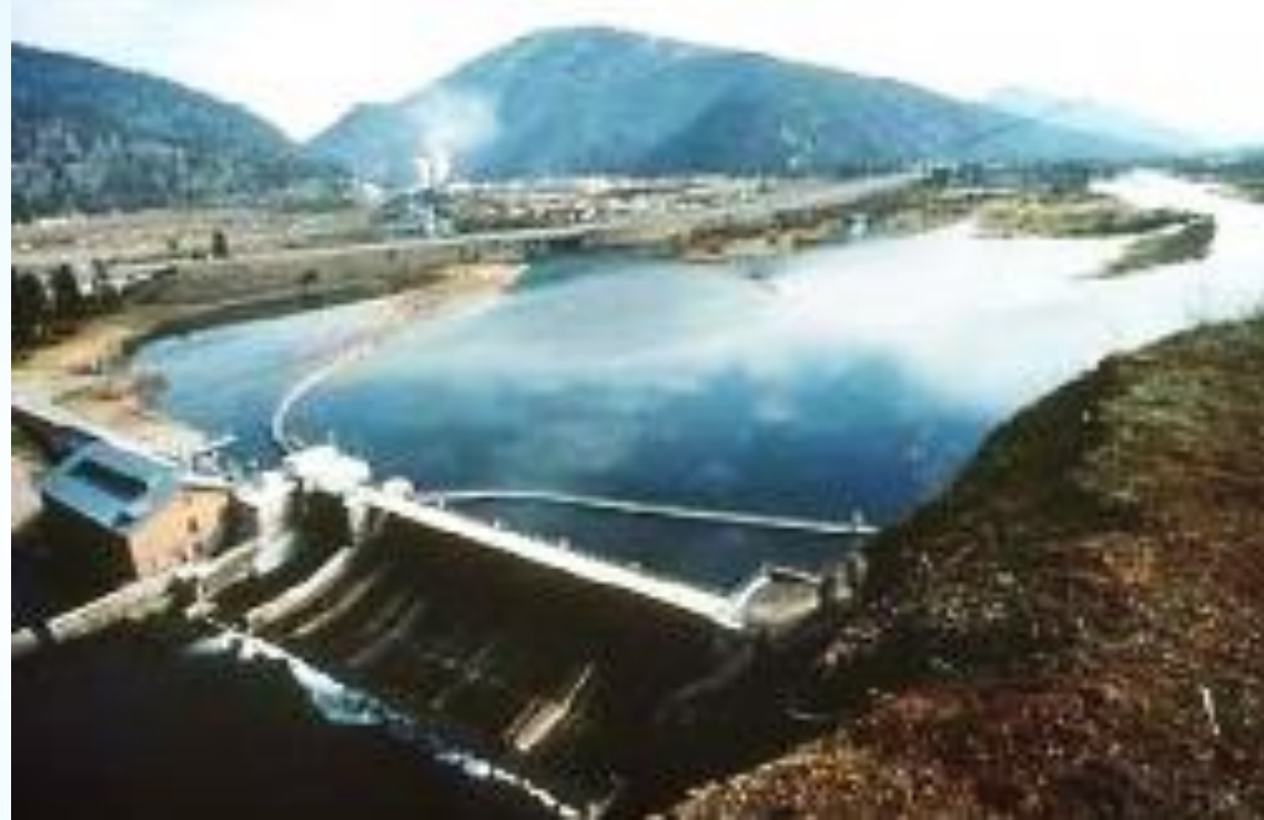
Milltown Dam, MT
