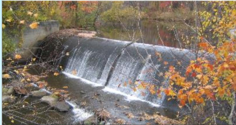
Engineered - Heminway Pond Dam, CT
