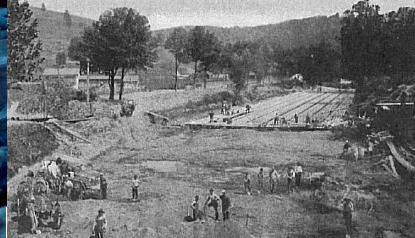
Cooling Pipes for Gas Pumping Station Under impoundment
