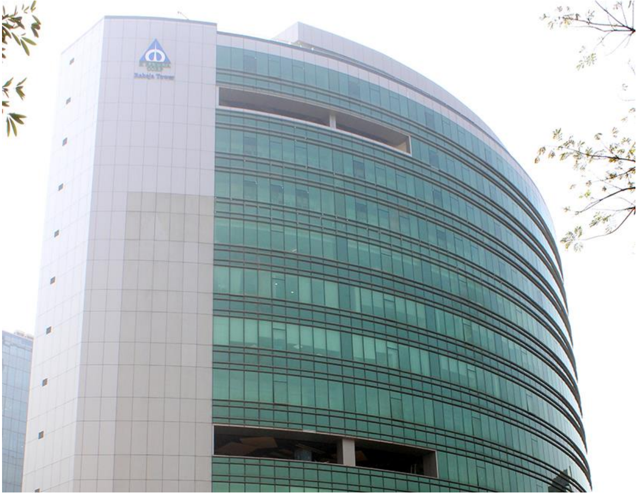
FIGURE 26 EXISTING CONDITION OF THE RAHEJA TOWERS
