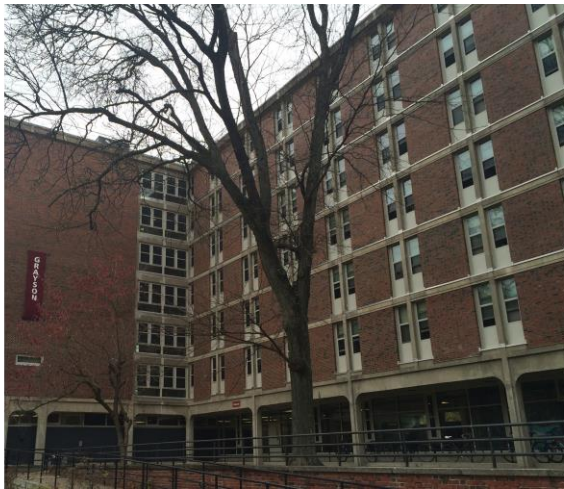
Figure 1: Grayson Hall west façade open windows. concrete.
