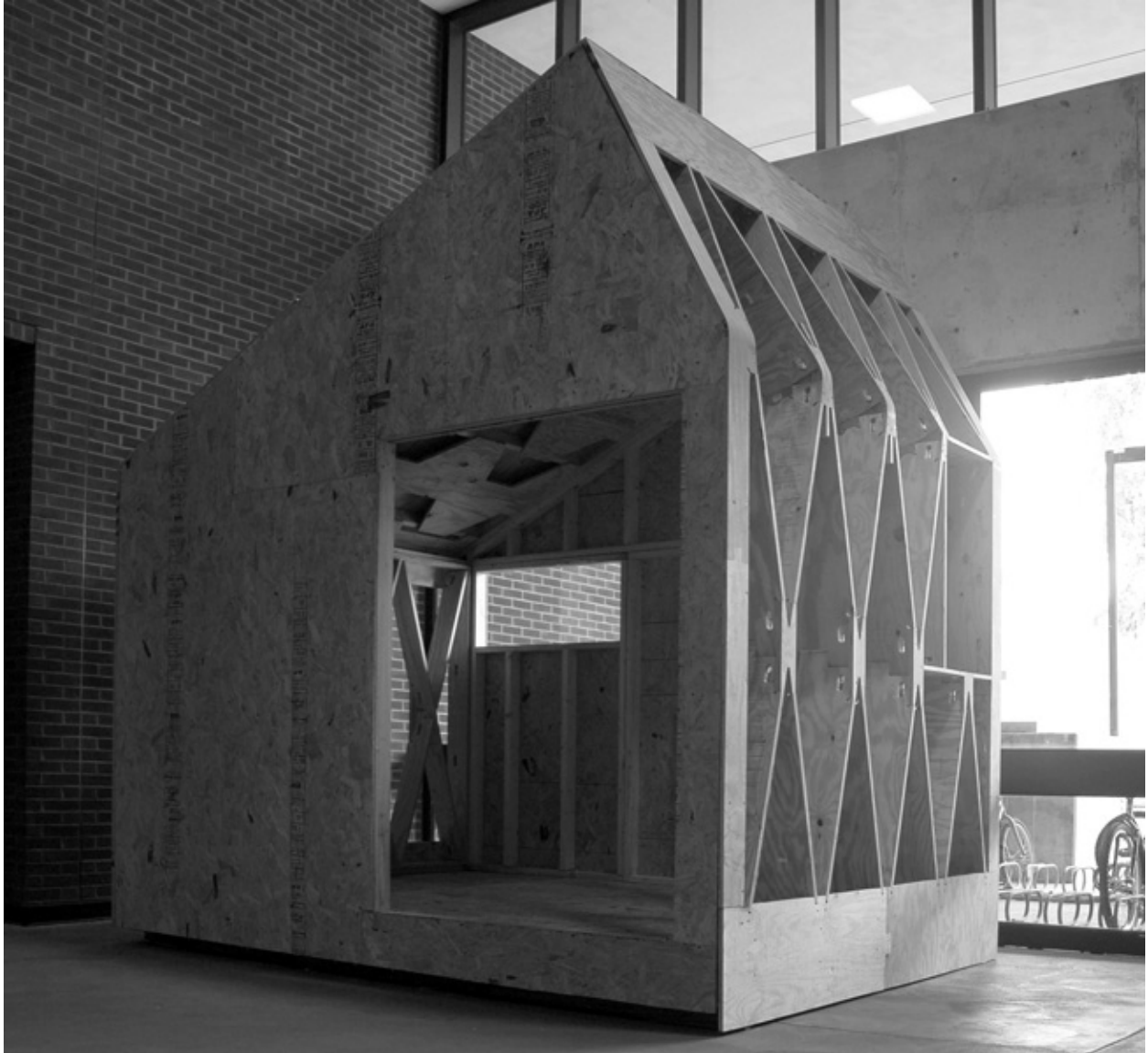
Fig. 3. Completed lattice-frame mock-up, showing all systems demonstrated at full scale
