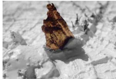
39 Detail of pulled wood, rotting log.
