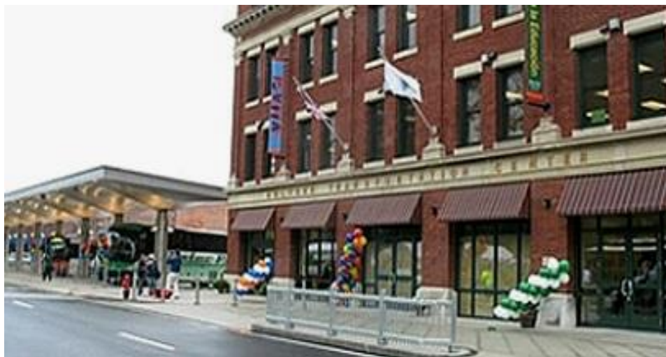
Holyoke Transportation Center. Source: PVPC
