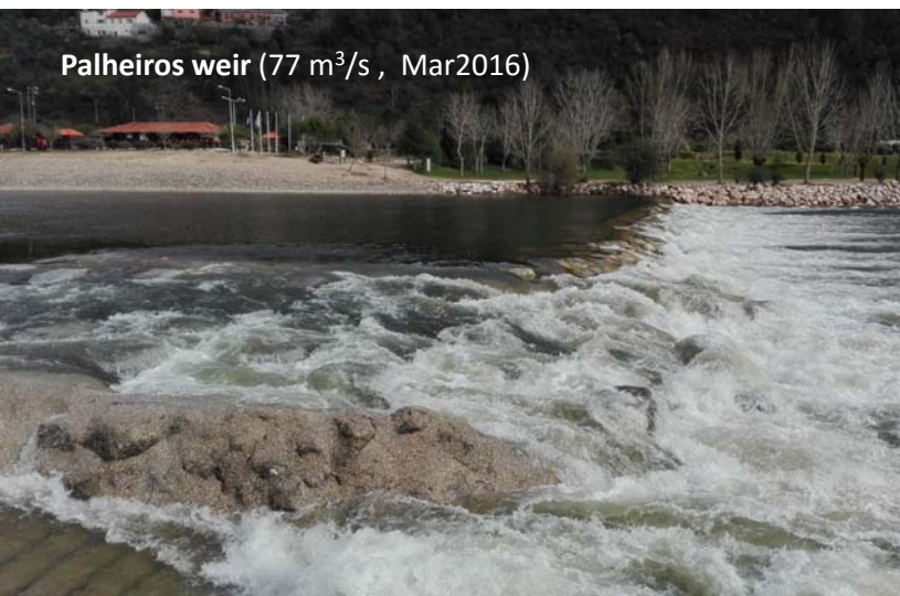
Palheiros weir (low flow condition / Sep2015)
