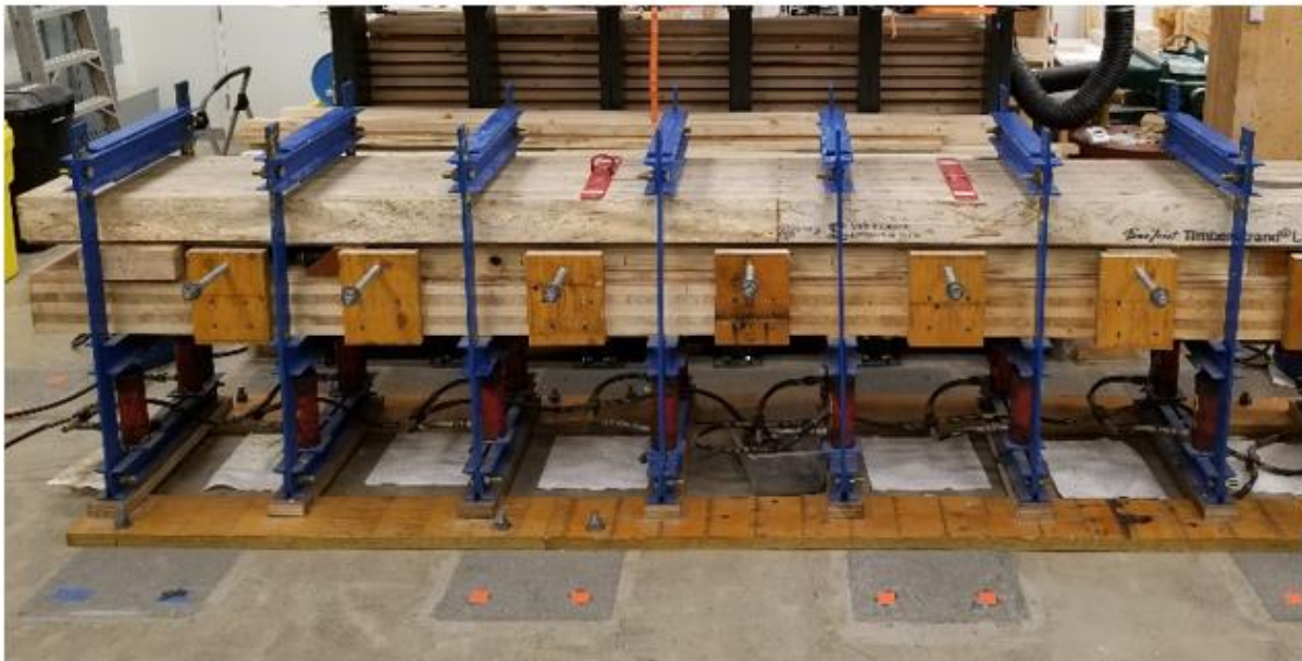
Figure 4.2: Fabrication process for short-span CLT panels
