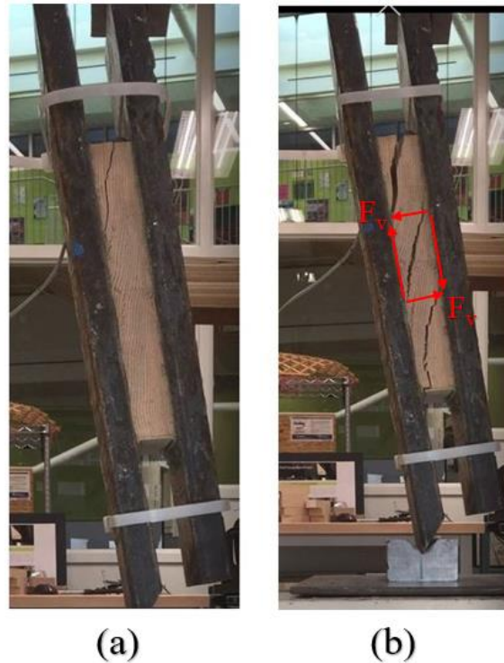
Figure 3.8: Failure mode I: (a) formation of the first crack (b) propagation of cracks along growth rings at final failure
