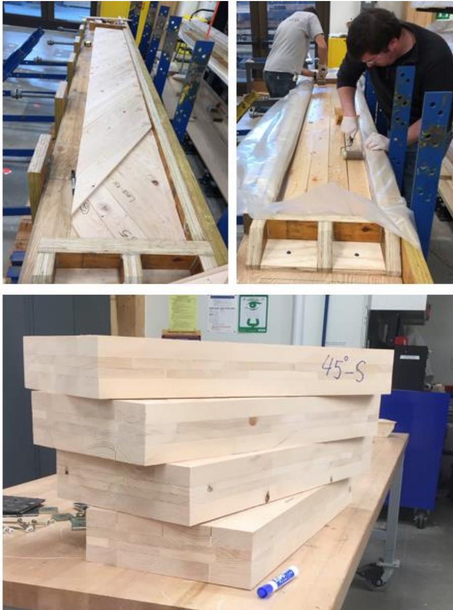
Figure 5.3: The detailed fabrication process for short-span CLT panels
