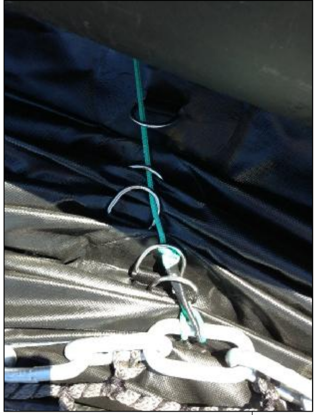
Pacific Netting Products Inc Iron Gate Dam Algae Barrier Typical Barrier layout Date: 1/15/2015 Drawn: PC-IGD-004 Rev: 0 Scale: None Not For Construction
