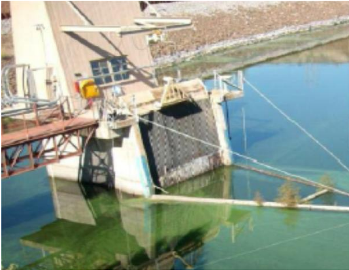
Iron Gate Reservoir Intake Tower, Trash Rack, and A-frame Debris Boom. (Photo Date: September 10, 2008.)
