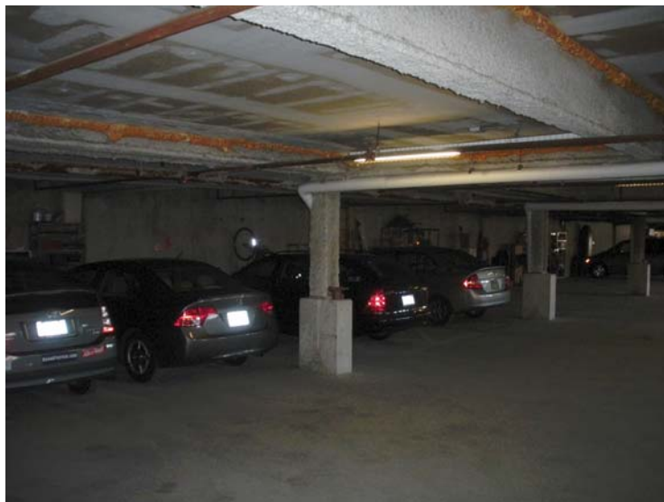
Figure 22: Underground Parking Garage
