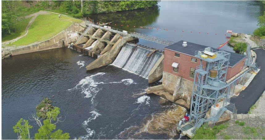
Figure 8. Scotland Dam Generating Station (41.6634° N, 72.1229° W) illustrating spillway, powerhouse, and fish lift tower (right). Image Credit: FirstLight Power Resources
