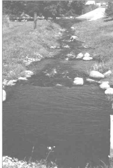
Figure 2. Pool and riffle nature-like fishway in Manitoba, from Katopodis et al 2001.
