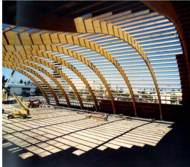
116' Span Anaheim Ice Arena
