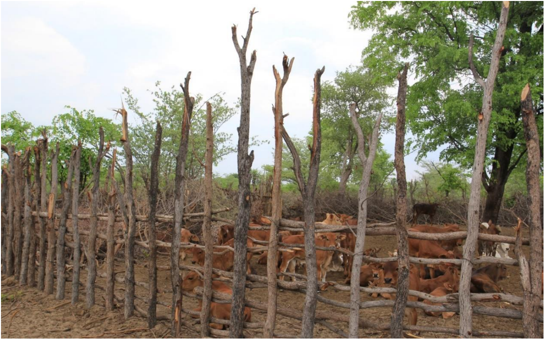
Figure 2.2. Traditional kraal structures in northern Botswana. A: thorn branch style construction, B: thick wooden branch construction. Photos by E. LeFlore.
