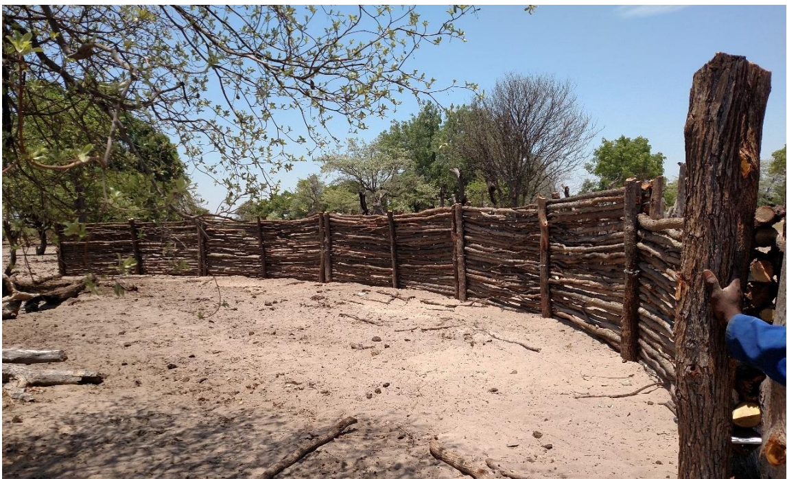
Figure 4.3. Pride in Our Prides newly constructed predator-proof kraals in the lion conflict study area in northern Botswana. Top: Rectangular woven mophane branch kraal. Bottom: Portion of circular stacked mophane trunk kraal.
