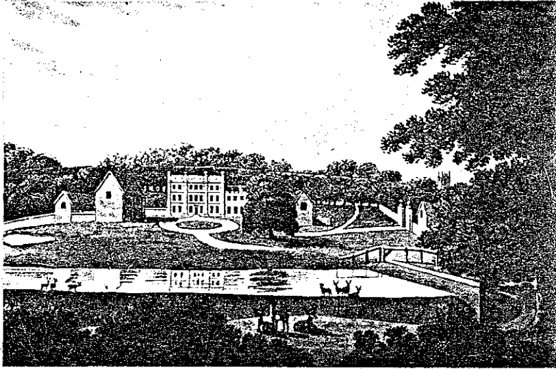
Fig. 25. South front of Harlestone Park before improvement.
