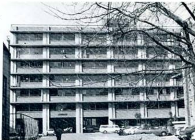
Faculty of Engineering, Hall 5, Applied Chemistry Departments
