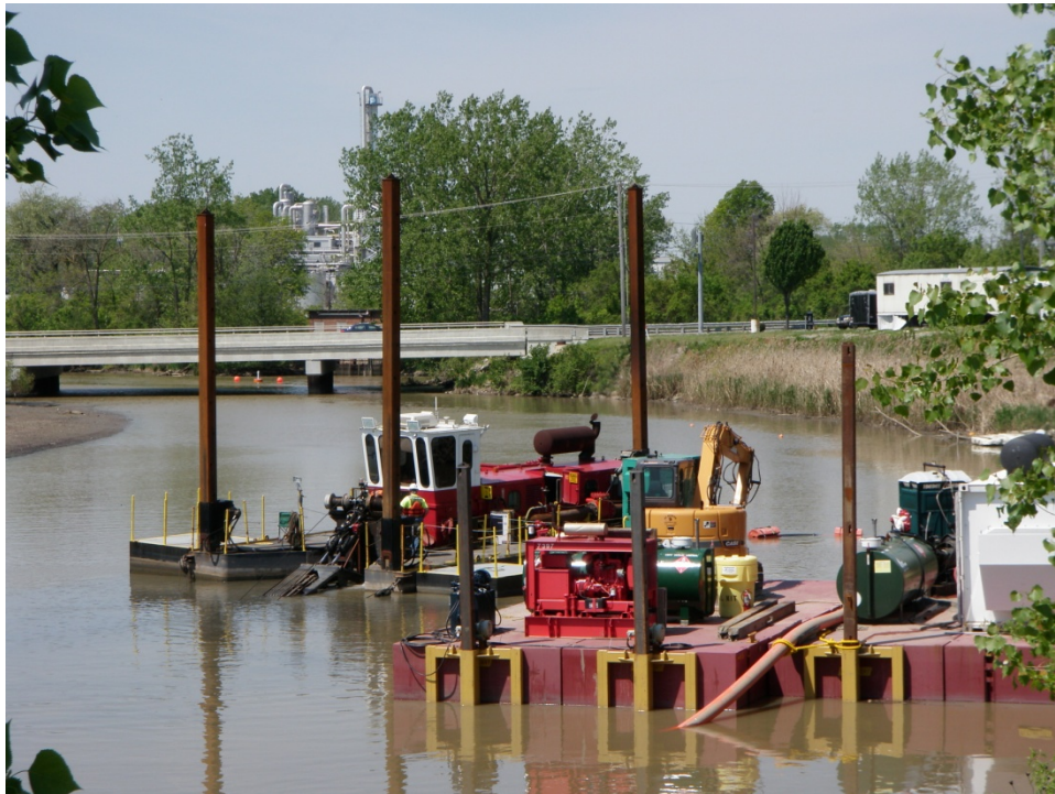
Figure 2. Ten-inch hydraulic dredge working area in Reach 2
