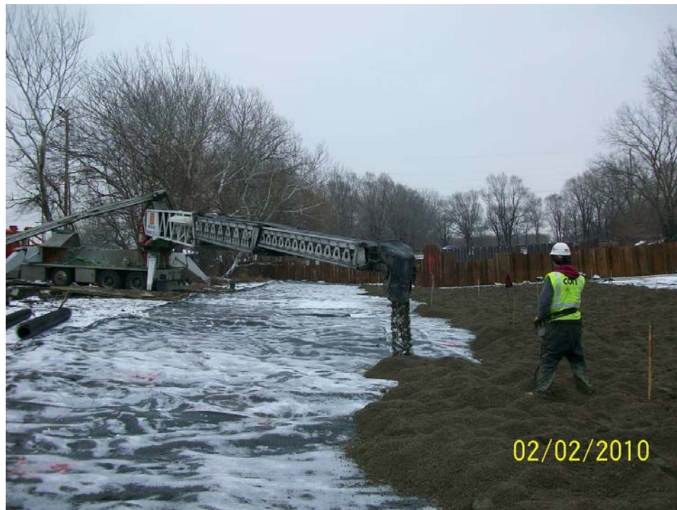
Figure 1. Granular cap placement by belt conveyor
