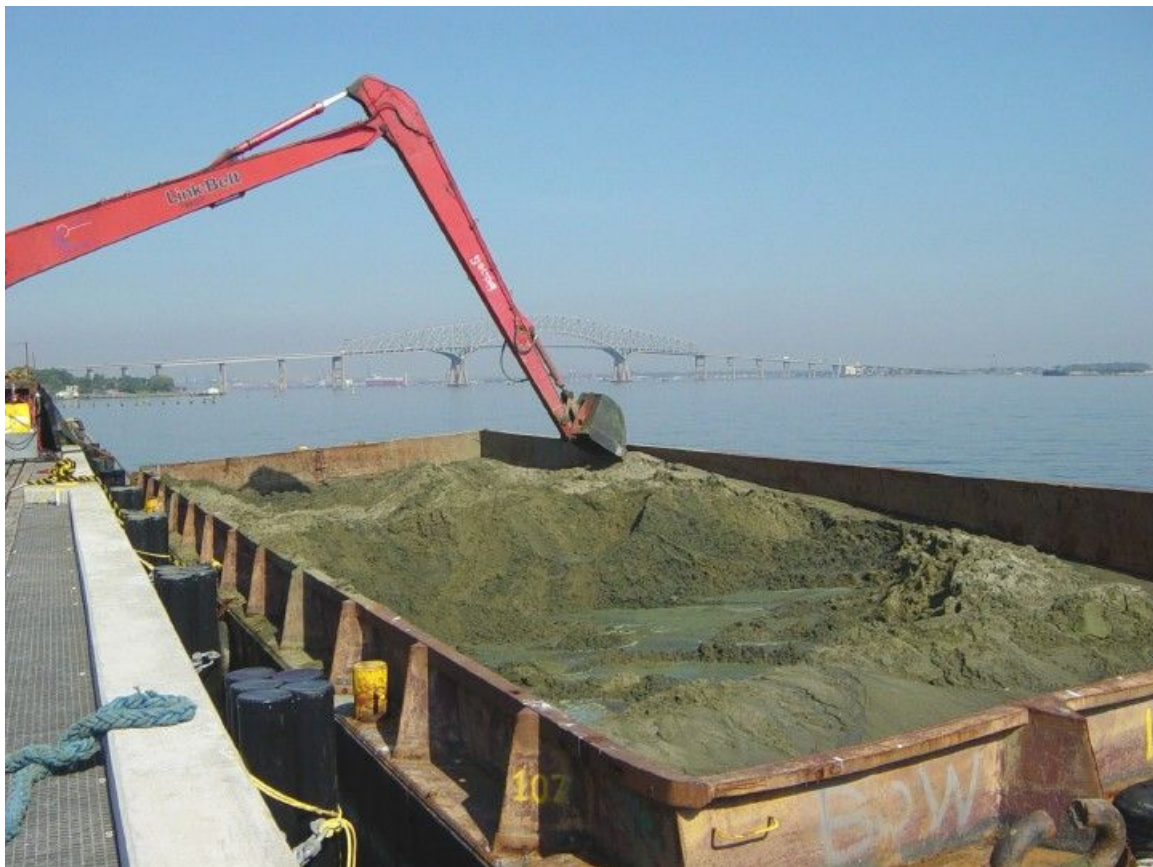
Figure 2. Cox Creek CDF Barge Unloading
