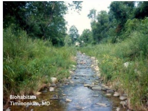
Figure 6 - Timonium, MD storm water channel - After
