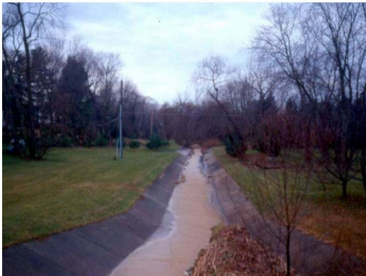
Figure 5 - Timonium, MD storm water channel - Before
