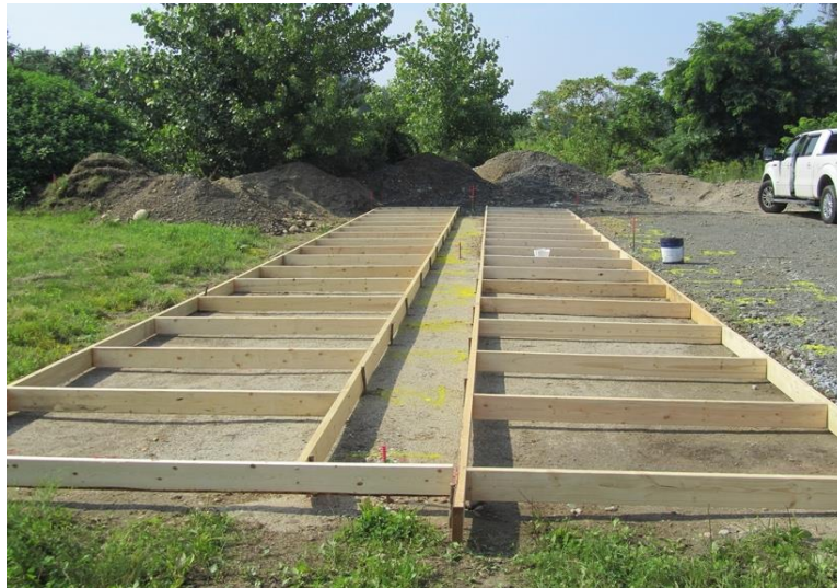
Figure 5.2 Panel groups D to I (looking south) with framing before placement
