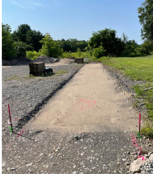
Figure 5.1 Panels groups A, B, and C after excavation (looking south)
