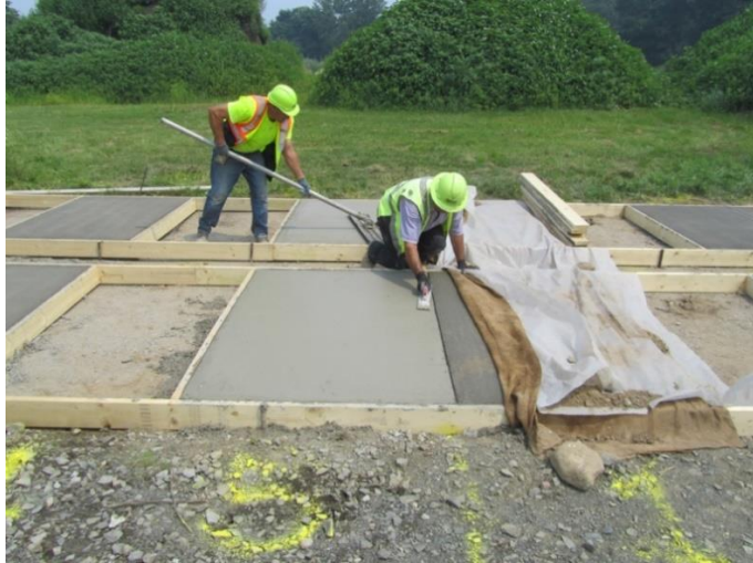
Figure 5.4 Workers use bull float and trowel on sidewalks
