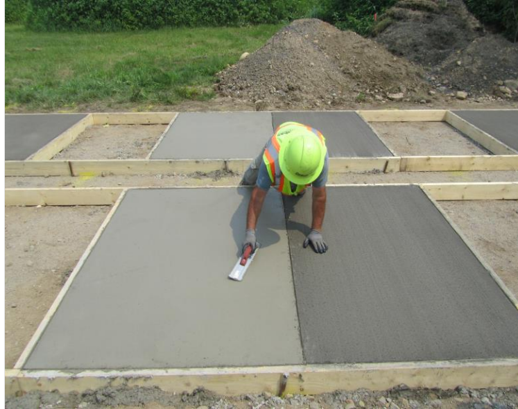
Figure 2.2 Worker trowels sidewalk panel following MassDOT specifications
