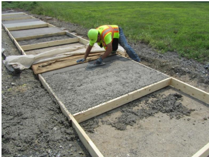
Figure 5.5 Worker uses trowel on concrete panel
