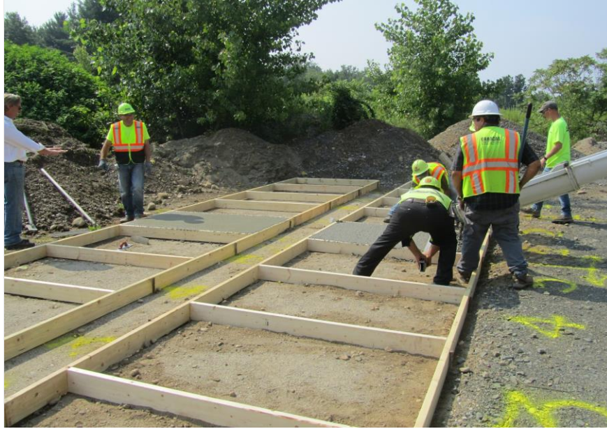
Figure 5.3 Concrete coming down the chute of concrete truck into panel frame
