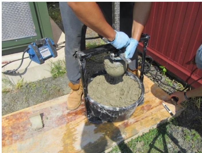
Figure 4.1 Project worker performing Vibrating Kelly Ball test on the concrete
