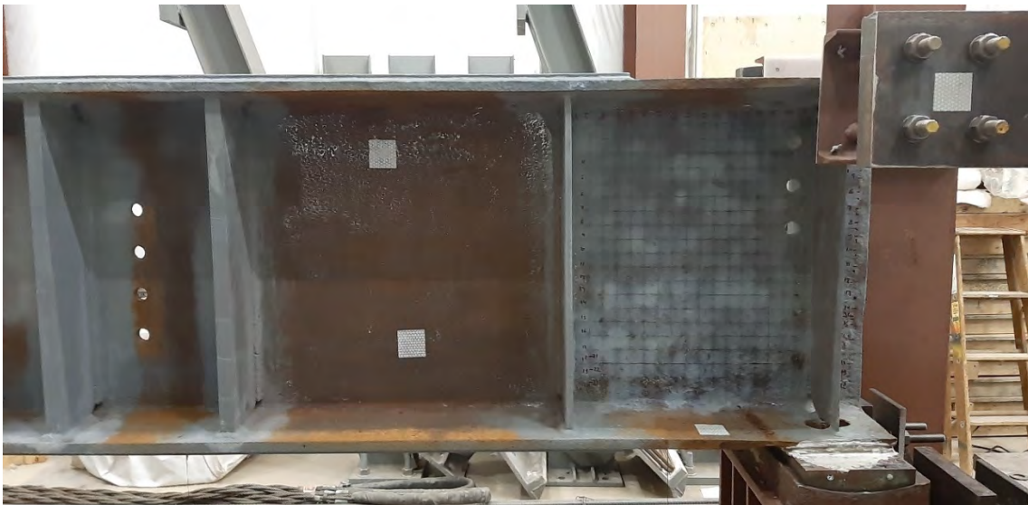
Figure 3.7: Corroded end of Specimen A
