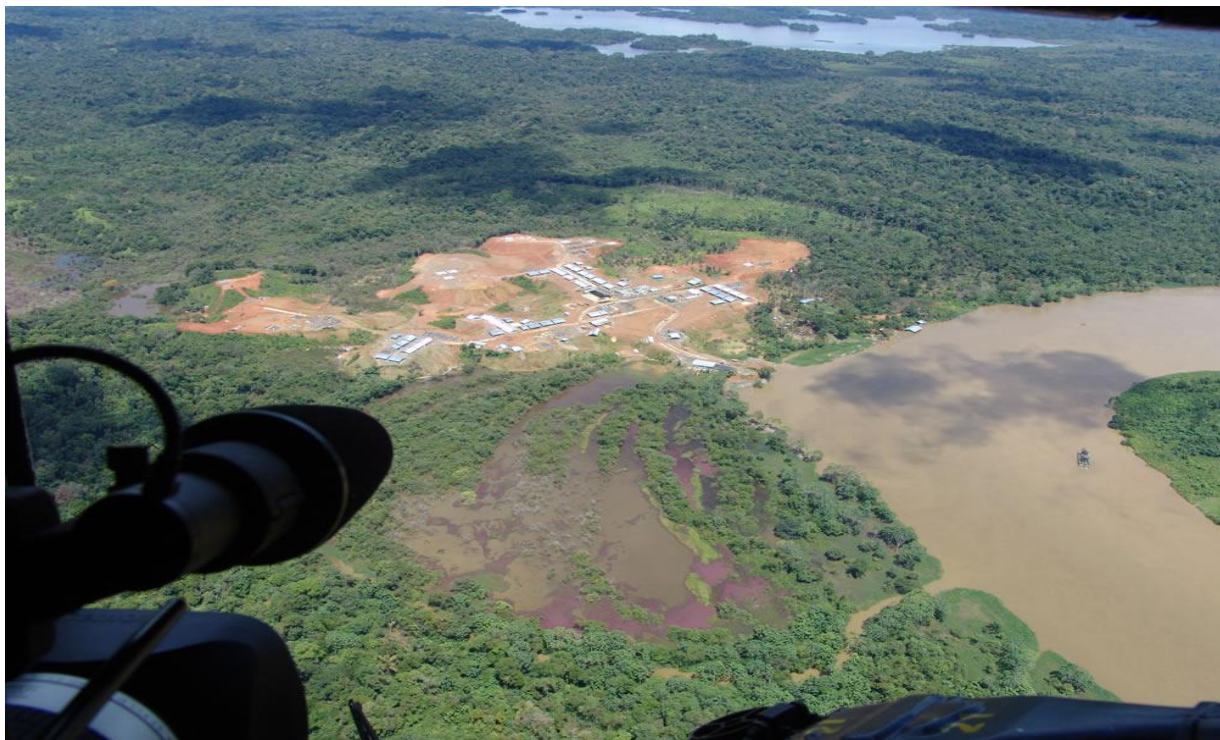
Figure 15: Aerial picture of New Bellavista- and Old Bellavista-Bojayá II, Acción Social
