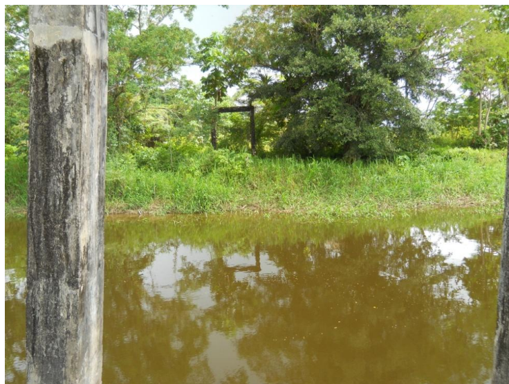
Figure 17: Destroyed Structure of the Brigde over the 'Caño'
