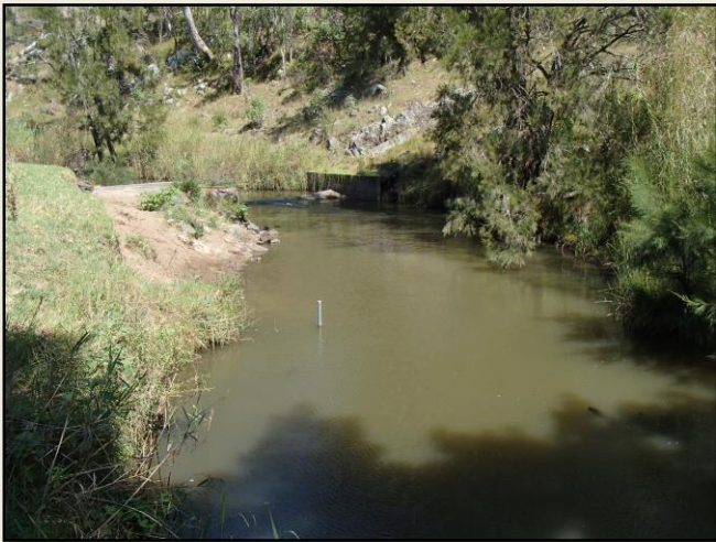
Elbow Valley Weir, Condamine River
