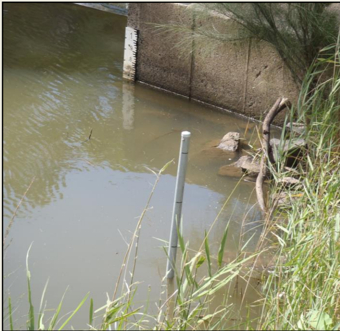
Upstream logger pole, Elbow Valley Weir, Condamine River, Queensland.
